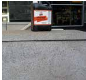
Result after leaving FPFO on overnight. Needs one more application to perfect
