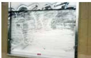
**TIP 2** A small amount of BARE BRICK, STONE AND MASONRY REMOVER (BBSM) can be added to SSR to increase the effectiveness and speed of the removal of some stubborn spray can paints on painted surfaces. This can be especially helpful in cold weather if SS appears to be a little slow. Work quickly, and on small areas at a time, to avoid any damage to the underlying surface. The use of a Scotch-Brite scourer is definitely of help in this instance to increase the removal speed.
